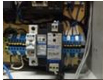
Electrical industrial boiler control, installed current sensor.
