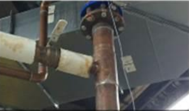
Hot water tank output, installed temp sensor
