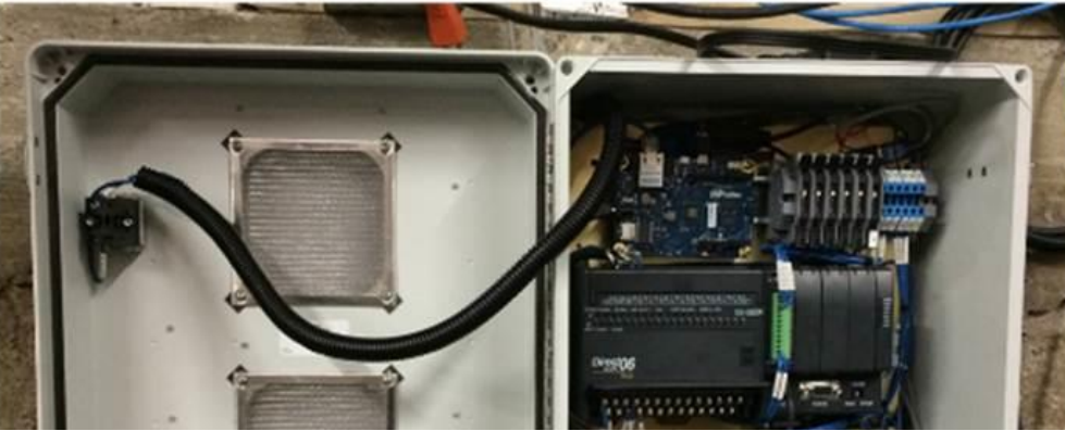
Dual water pump system with digital control, installed current sensor.
